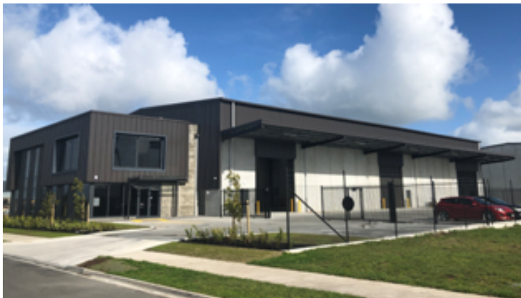
During the year, Chalmers Properties embarked on a new design/build/lease development for NZ Windows (Waikato) Ltd at 25 Clem Newby Drive. The building is the largest build to date at Te Rapa Gateway. Situated on a 3323m 2 site, it comprises 1305m 2 of warehouse, 378m 2 of office space and a 270m 2 canopy.
