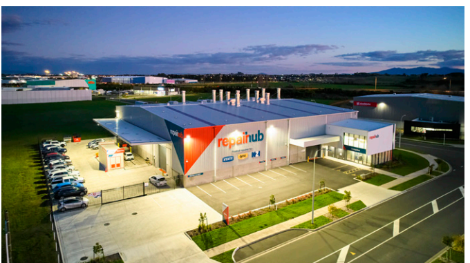
Completed in January 2022, the IAG Repairhub was the first DBL for the client. The 2245m 2 office/warehouse development won a Merit award at the 2022 Property Industry Awards.
